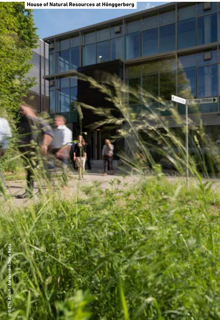
House of Natural Resources at Höggerberg
